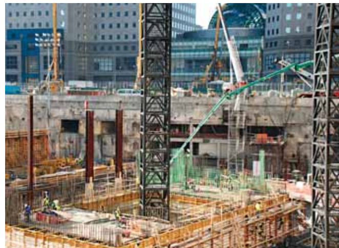
PHOTO: JOE WOOLHEAD, COURTESY iCRETE
