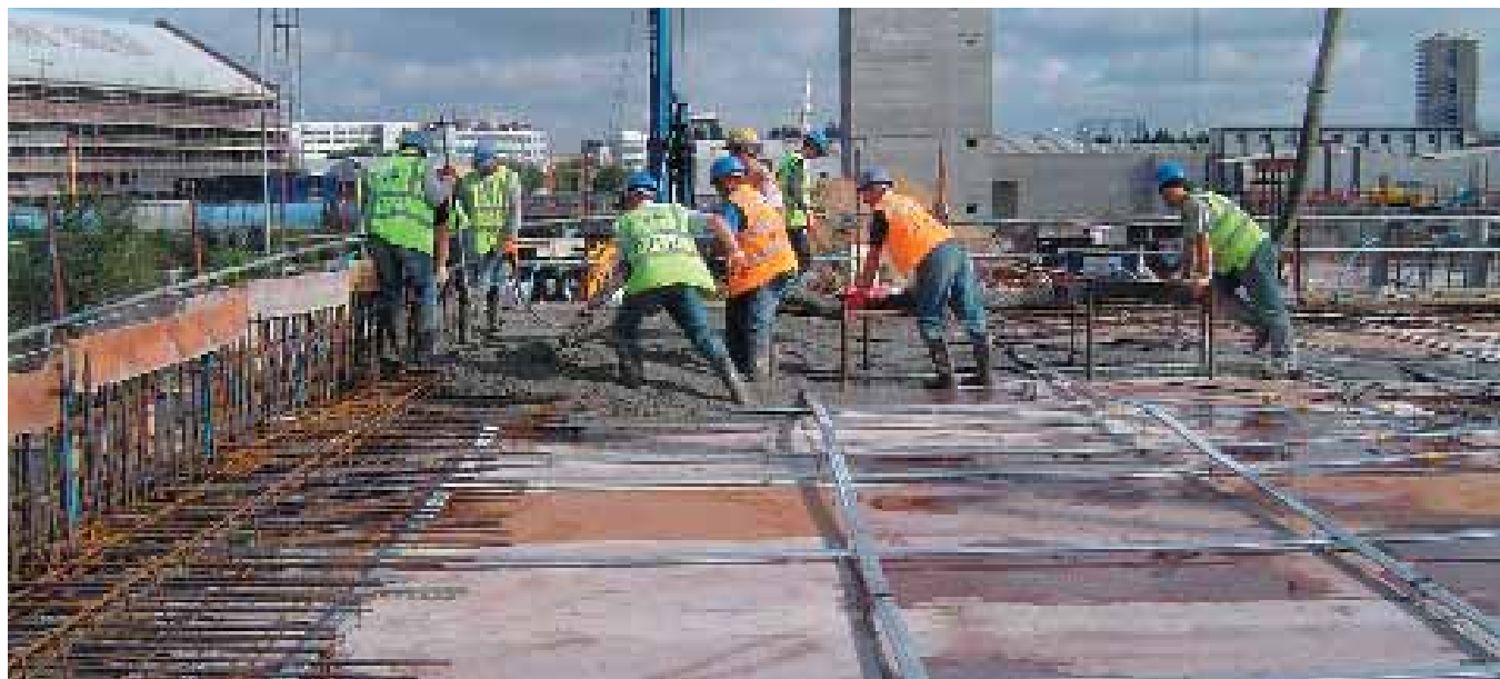
A post-tensioning process underway: New techniques in post-tensioning include the use of intumescent materials in the post-tensioning process to increase the fire resistance of concrete structures.
