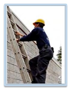
In the photo above, the worker is safe because the base of that 20 foot ladder is 4 feet (or ¼ of the working height) away from the 16 foot wall.
